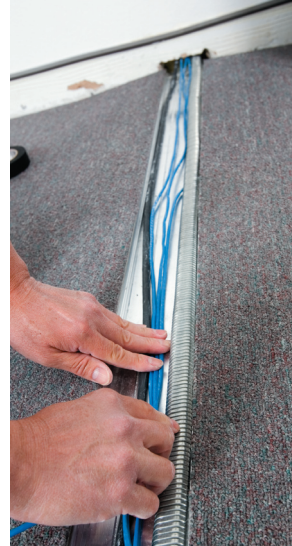
Ensure cables lay flat
